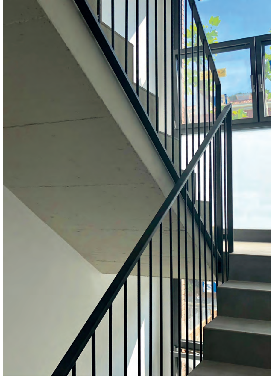
Interior residencial FERRO BLOC
