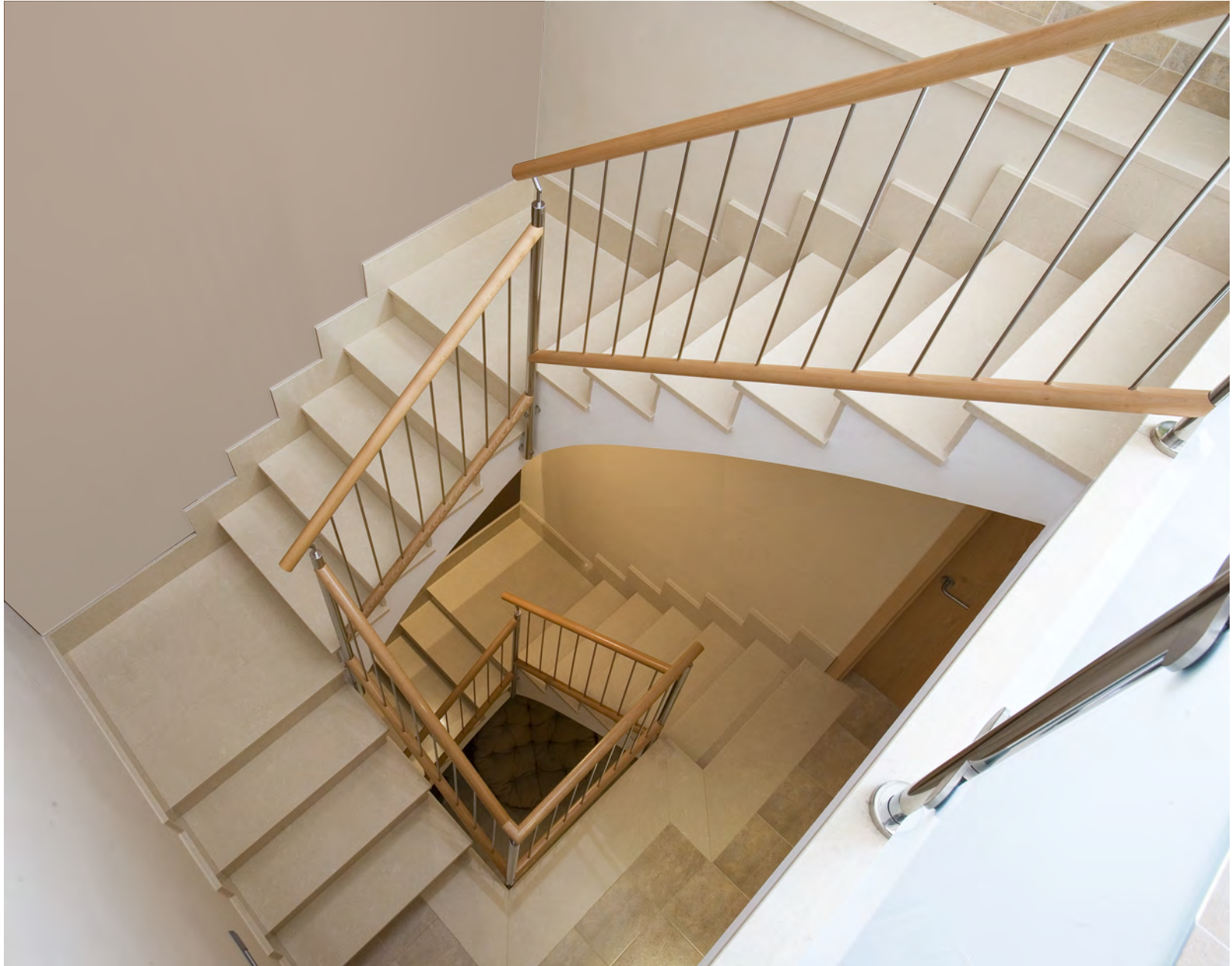
Interior residencial INOX-6
